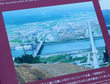
気仙川にかかる希望のかけ橋。主塔間距離220mの長距離ベルトコンベア専用の仮設橋でした。 The Dream Bridge over the Kesen River. It was a temporary bridge dedicated to connect long distance belt conveyors with a distance of 220m between its main towers.
