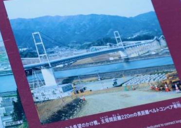
気仙川にかかる希望のかけ橋。主塔間距離220mの長距離ベルトコンベア専用の仮設橋でした。 The Dream Bridge over the Kesen River. It was a temporary bridge dedicated to connect long distance belt conveyors with a distance of 220m between its main towers.
